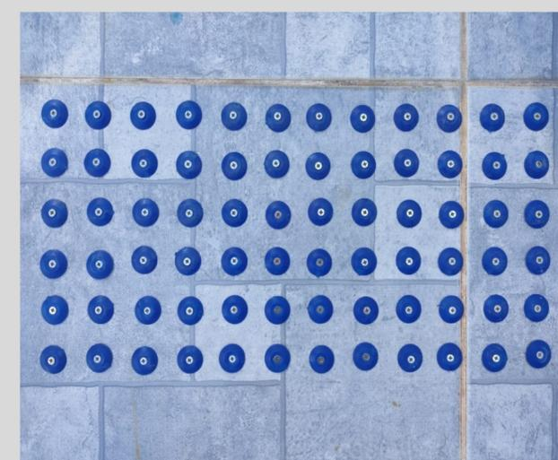
FOTO ILUSTRATIVA DO RELEVO TÁTIL PVC DISCREET ALERTA FIXADO COM BUCHAS E PARAFUSOS - ÁREA EXTERNA
